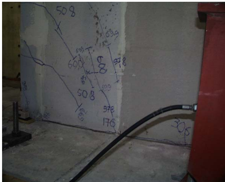
Figure 6.26 View of North compressive toe of Shear Wall Specimen 17
