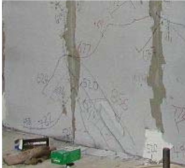
Figure 6.29 Diagonal cracks around the dowels of the assemblage specimen
