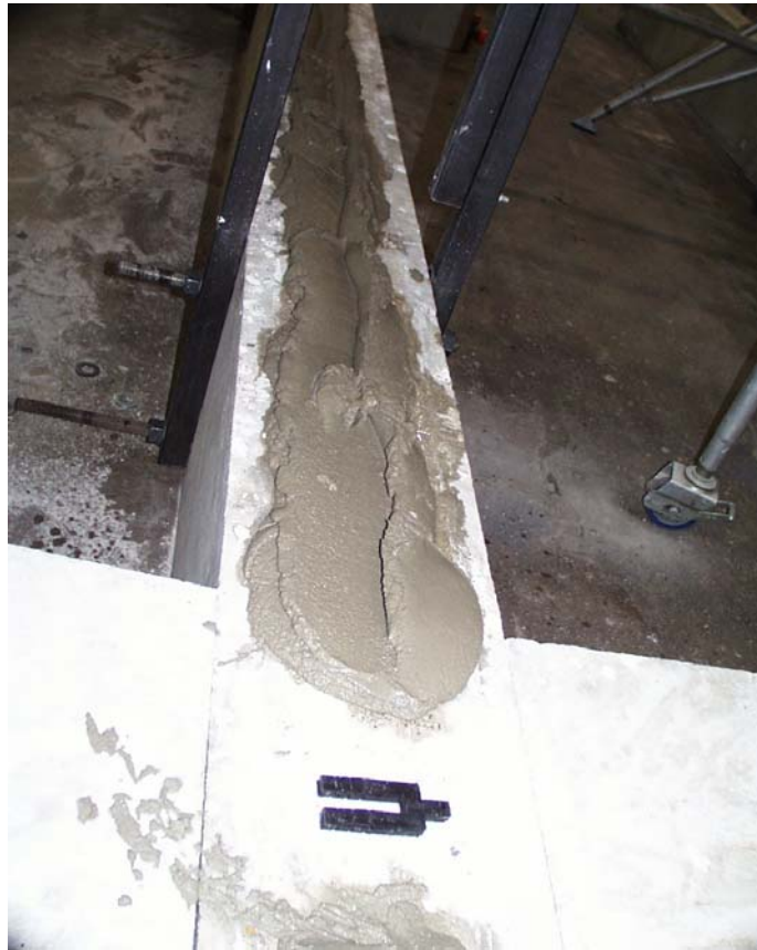
Figure 2.3 Placing Type S mortar by proportion on concrete foundation
