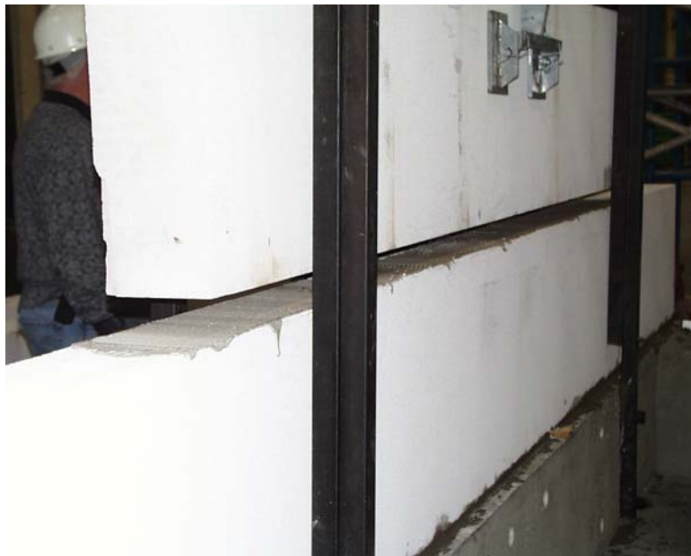
Figure 2.5 Placing second course of AAC panels
