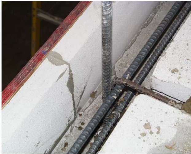
Figure 135: Photograph of Detail A, at intersection with vertical bar
