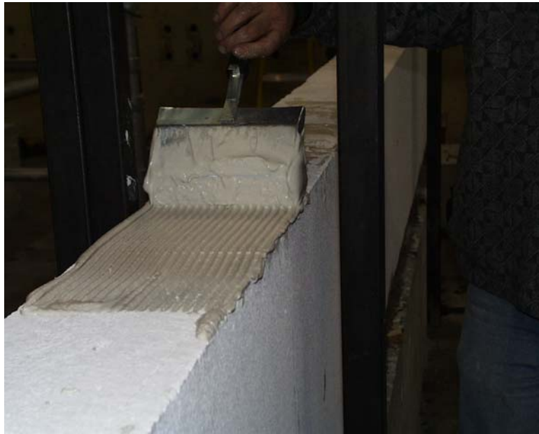
Figure 2.4 Placing a layer of thin-bed mortar on AAC panel
