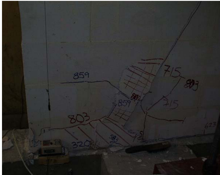
Figure 5.24 Crushing of the north compressive toe of Shear Wall Specimen 7
